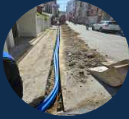
Placing Microduct
