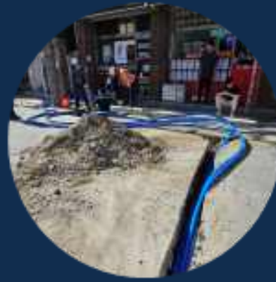
Microduct on curve
